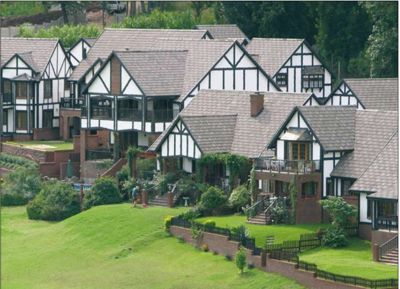
Windsor Crescent, Cluster Houses, KwaZulu-Natal
