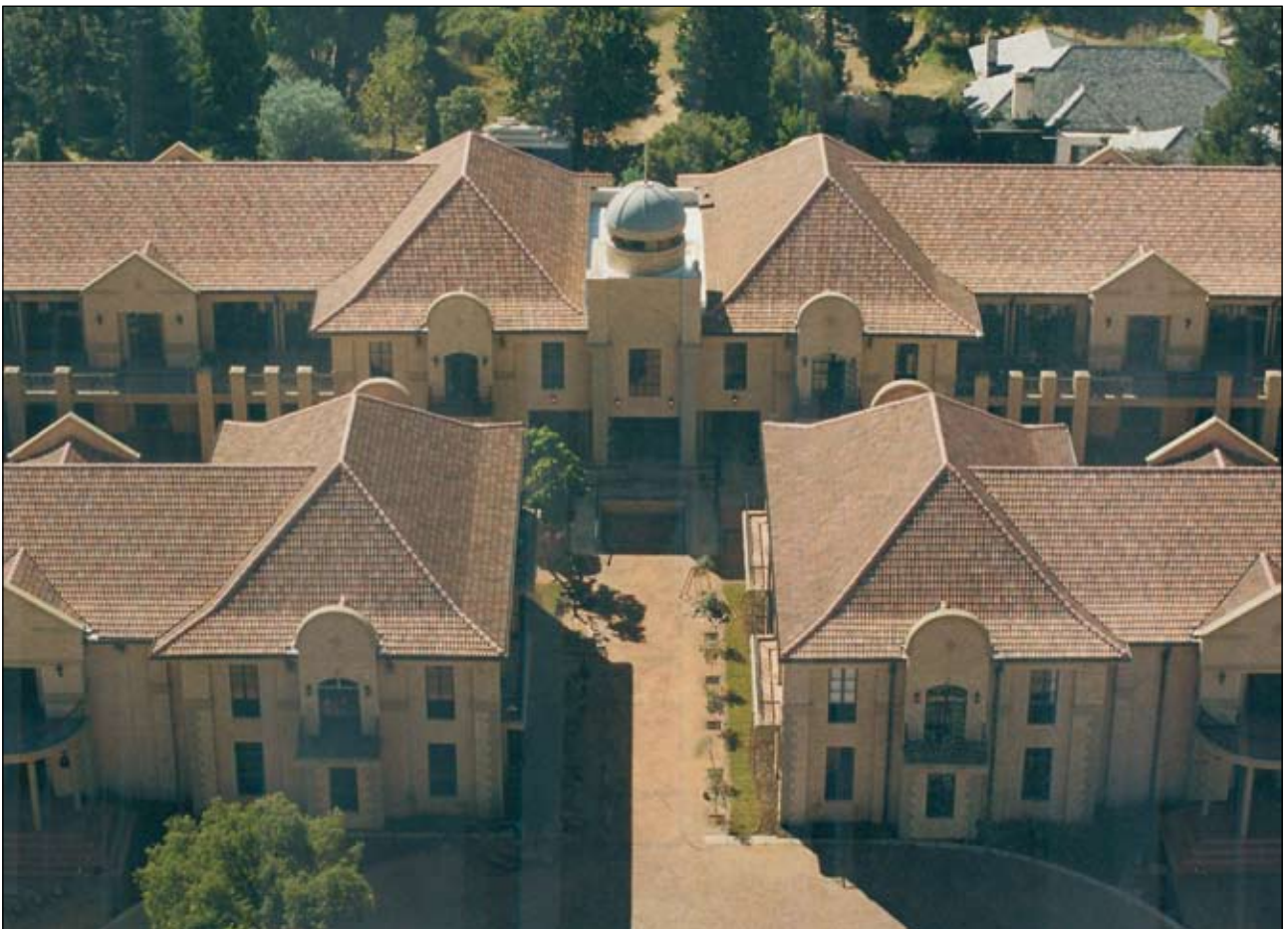
Bryanston Wedge, Office Development, Gauteng
