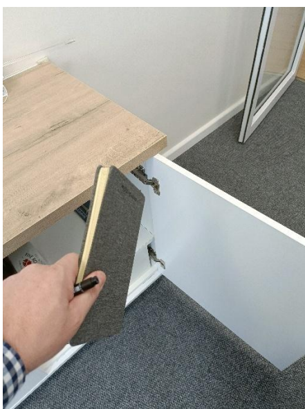
97. Loose hinge. The whole panel moves. Open up there door all the way. You will see the panels isn't inline anymore. Now press against it to level it out and then open the door again.
