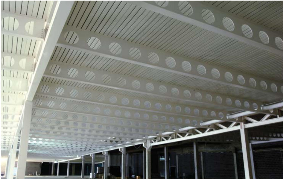
Car Park Structure
