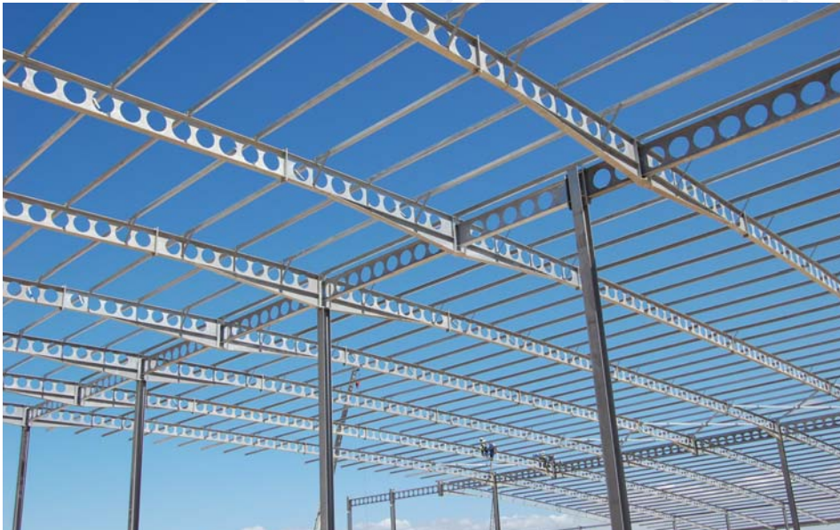
Cold Storage - Port Elizabeth
