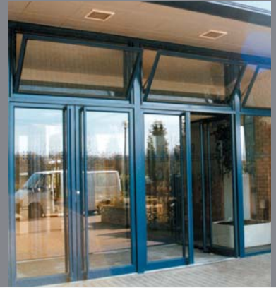
Shenley Pavillions, Milton Keynes. Automatic opening ventilators provide air inlet above the entrance doors.
