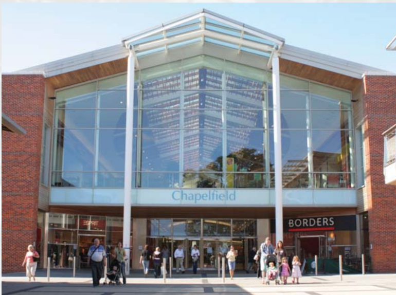
Chapelfield Shopping Centre, Norwich. Alongside a stairwell ventilation scheme, Seefire and Kameleon natural ventilators provide smoke ventilation for the malls and the House of Fraser anchor store.
