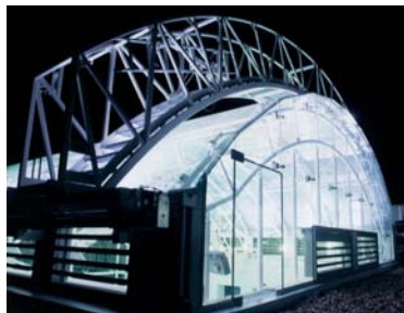
House of Fraser, Guildford. OPV controlled FCO Ventilators with polycarbonate louvres are installed at high level within the main glazed central atrium.
