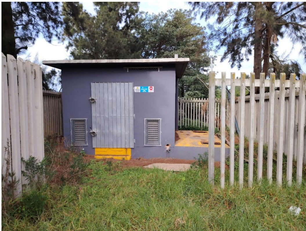
Figure 5: Existing Queen Street Pumpstation – Site Investigation 3 July 2024
