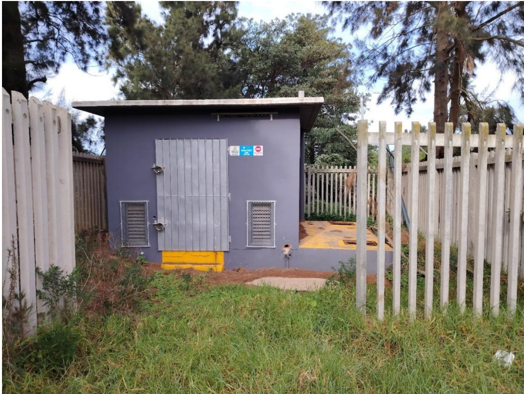
Figure 5: Existing Queen Street Pumpstation – Site Investigation 3 July 2024
