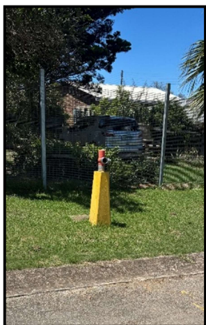
Figure 5: Existing Fire hydrant
